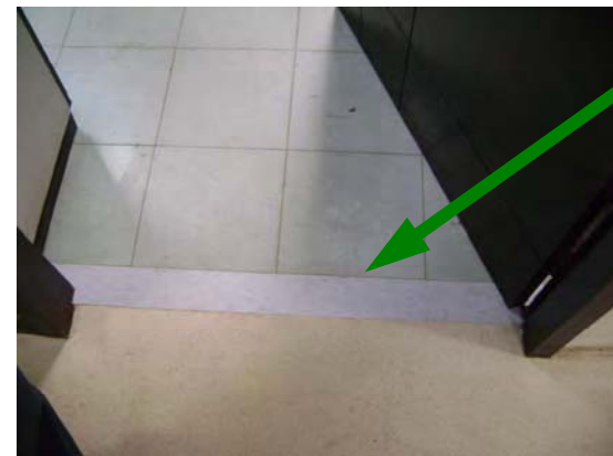
Record room entrance
