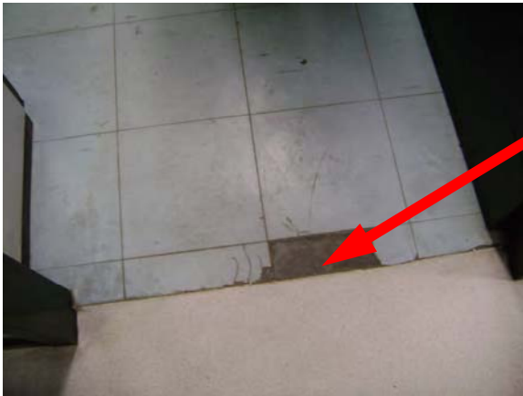
Record room entrance
