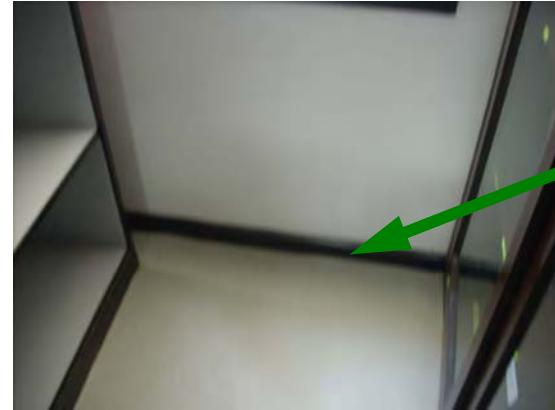
Items cleared on the gang way
